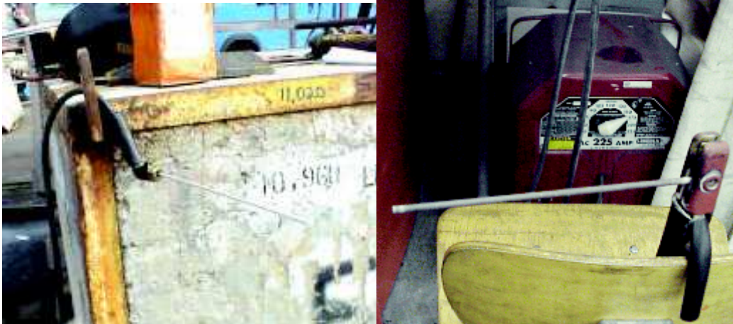
Figure 17 DANGEROUS CONDITION - Unattended Energized Electrode Holder
